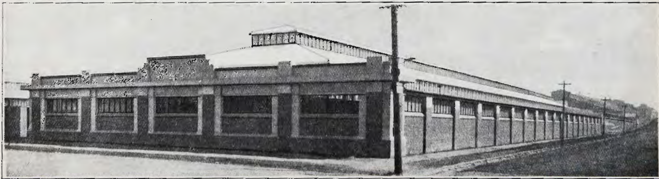
THE NEW HORSE PAVILION. Top: Back View. Lower: Front View, facing Public Street. Length, 345 Feet. Width, 105 Feet.
